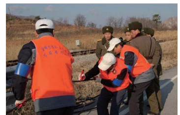
Construction to Upgrade inter-Korean Military Communications Lines
