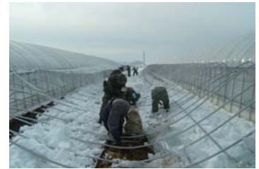
Supporting snowfall damage recovery (Dangjin, Chungnam, January 2009)
