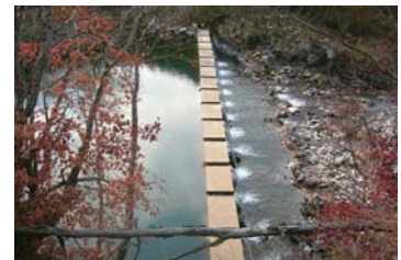
Regulating Reservoir Dam
