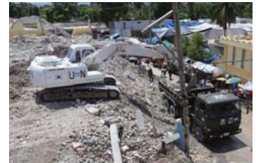
The Danbi Unit performing restoration work (June 2010)
