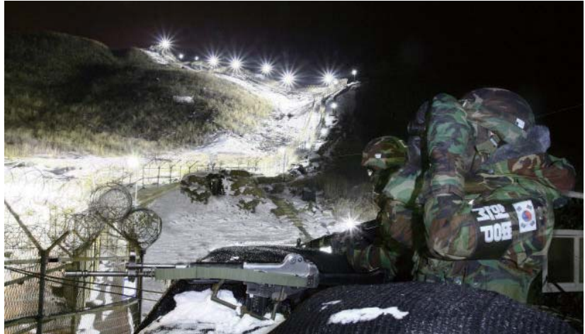
LED Lamp Installed on an Army GOP Barbed-Wire Fence
